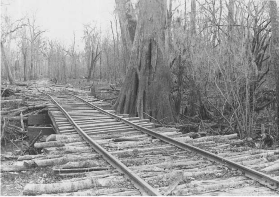
*Figure 4-5. A temporary railway laid for the extraction of cypress logs from the swamp (courtesy Glen Montz).*
